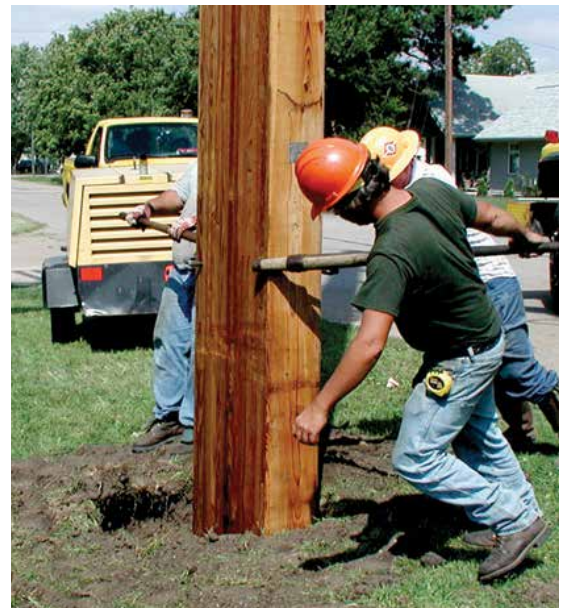
Adjust and align structure using a cant hook or similar tool.
