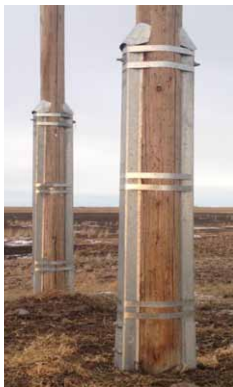
6. Units are banded and caps are installed.
