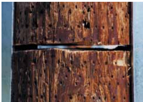
The pole is cut completely through.
