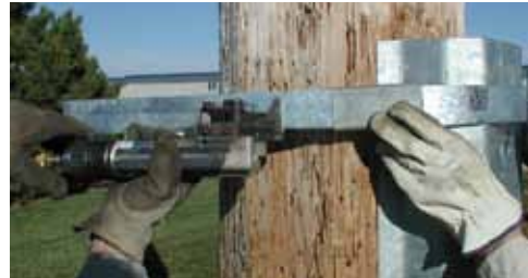
Tension the Banding using either an Air or Manual Tensioner.† Hit Banding with hammer to help tensioning.
