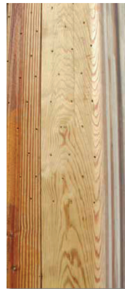
Groundline deep boring.
